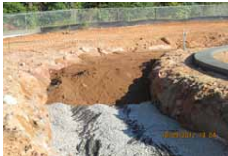
Soils high in organic matter and sand overlay the gravel which also increases infiltration.
