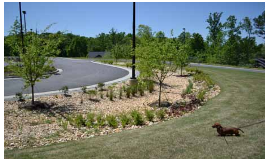
All impervious surfaces create stormwater during rainfall. Four features at the new Habersham County Judicial Center provide models of how to reduce the volume and the impacts of stormwater through better design, such as this “curbless bioswale.”
