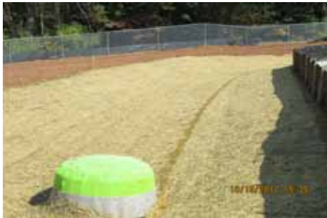
Completed construction of bioswale prior to vegetation.
